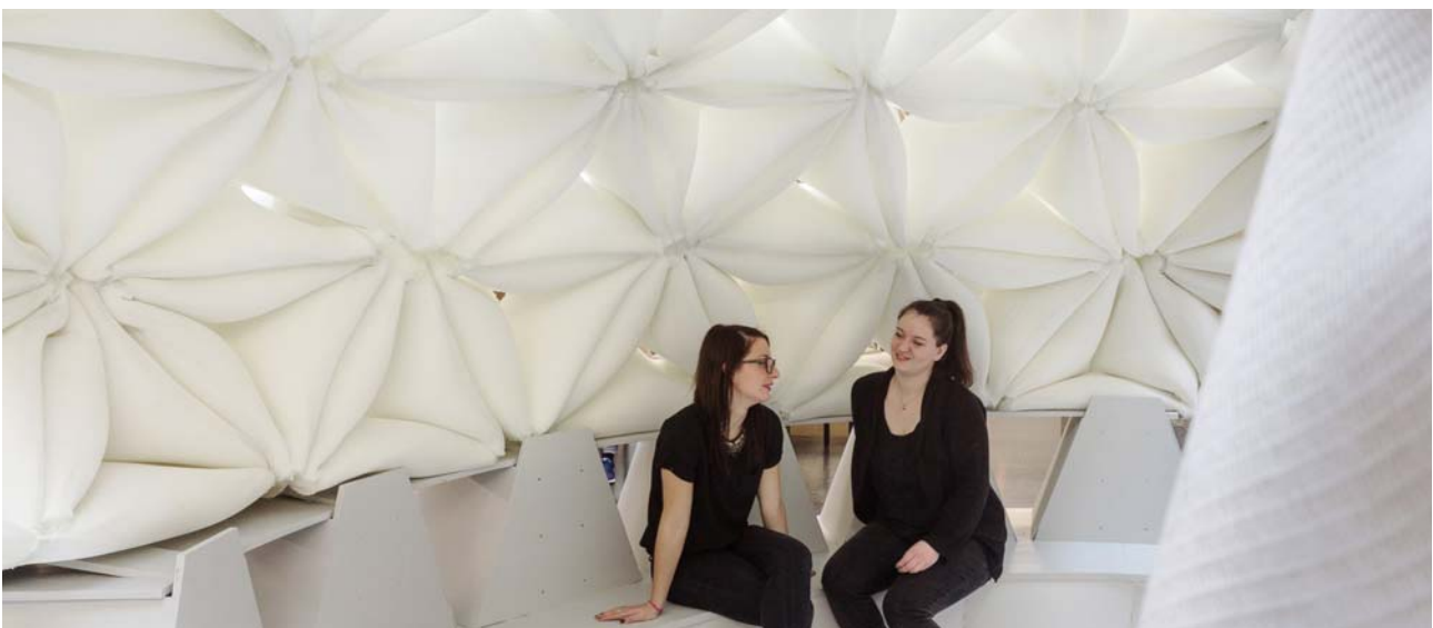
Partially foamed spacer fabrics for lightweight applications in architecture (Image: Tobias Etzer)
