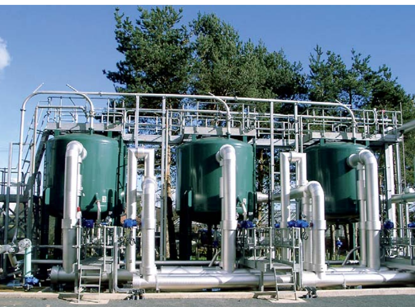
Figure 9: Fixed bed reactor system made of iron hydroxide pellets - Bayoxide® E33 – with very finely structured surfaces in the nanorange for arsenic adsorption (Source: Bayer AG, Severn Trents Services)
