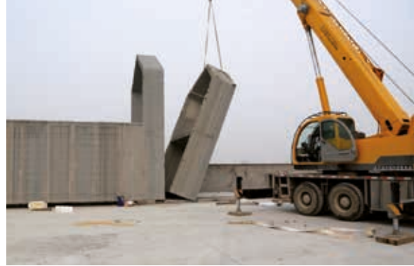
Erecting additively manufactured building components (Source: WinSun Decoration Design Engineering)
