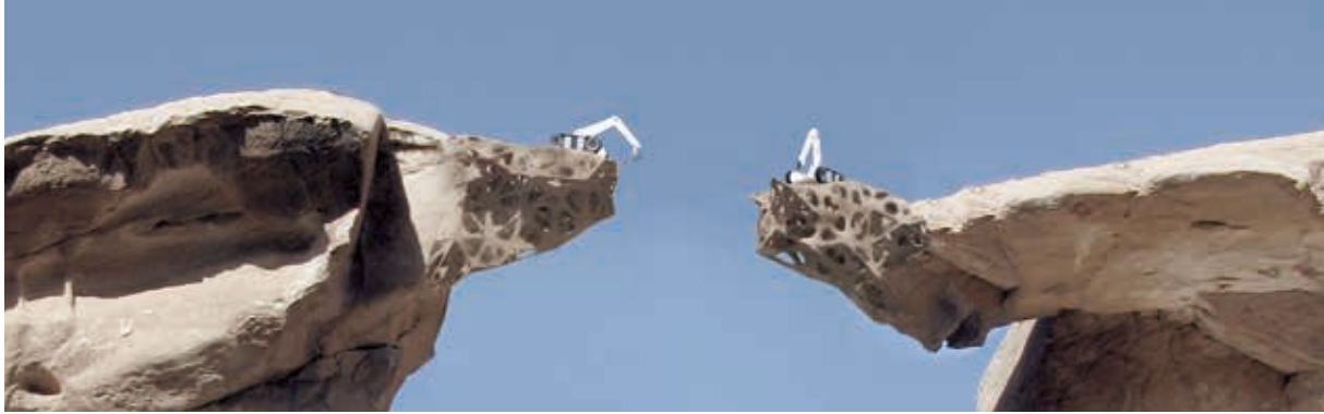
Stone Spray robots for bridge construction (Source: Anna Kulik, Petr Novikov, Inder Shergill)
