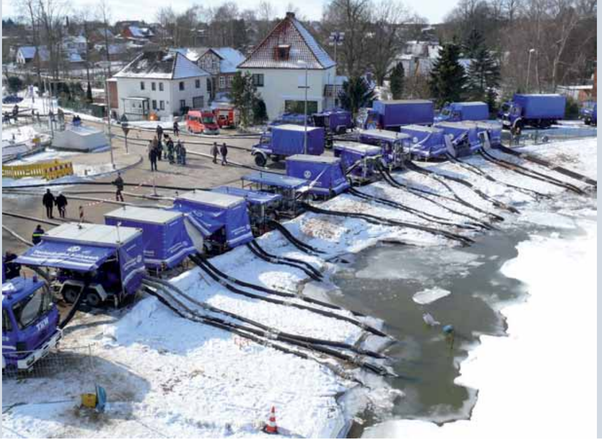
Pressure from melt water threatens to break a barrage. Source: German Federal Agency for Technical Relief (THW)
